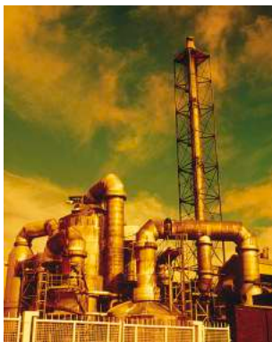
Figure 2: A sulfuric acid plant in Cleveland.
